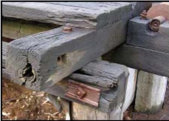
**Plate 28** – Detail of the south-western corner of the plank-saw bench, showing the evidence of recycled timber and repairs.
