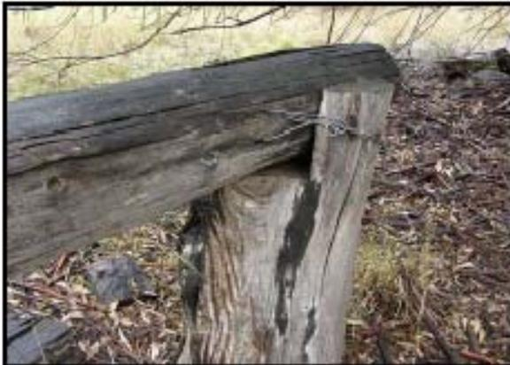
**Plate 46** – Detail of the fastening to the western end of the first log in the log rack.
