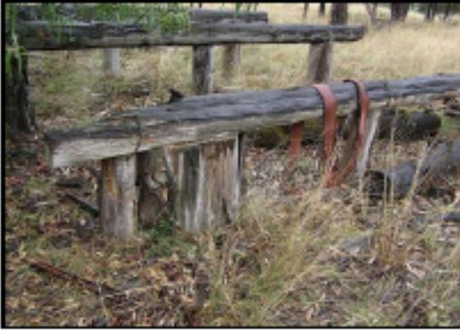
Plate 49 – View showing a large log placed under the damaged third log of the log rack.
