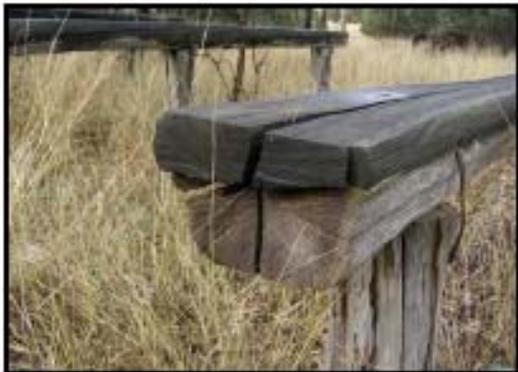
**Plate 53** – Detail of the end of one of the rails in the squared-log rail, showing that it was hand-sawn. Note also the flat top.
