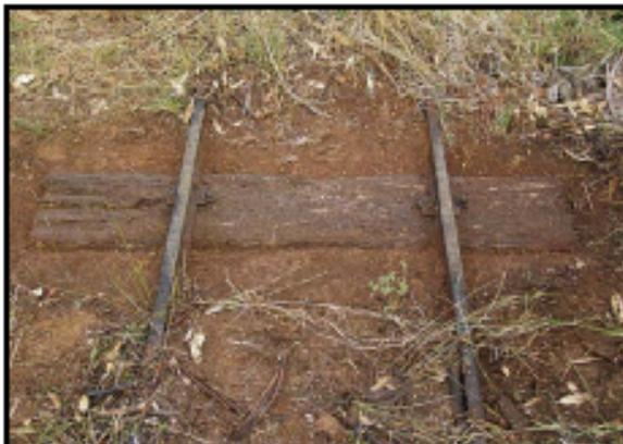
Plate 37 – A section of log-trolley track.
