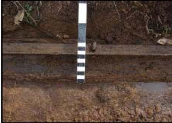
**Plate 43** – Detail of the plank-trolley track. The hook spike is clamping the flange of the angle iron to the longitudinal timber sleeper (scale segments 1 cm).
