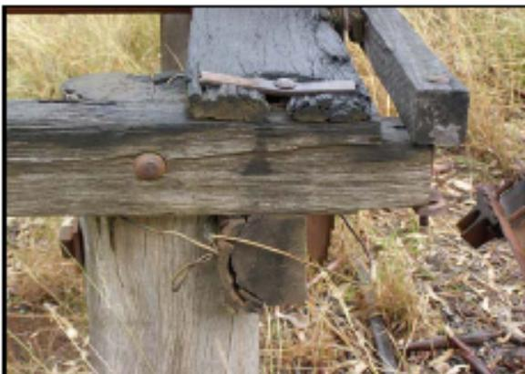
**Plate 12 – Detail of the repair work to the log-saw support frame.**
