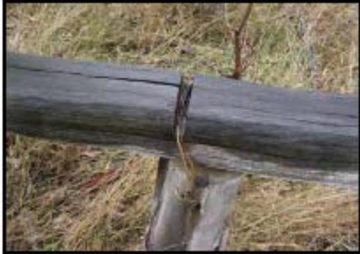
**Plate 52** – Detail of the fastening in the squared-log rack. Note the flat top to the rail.
