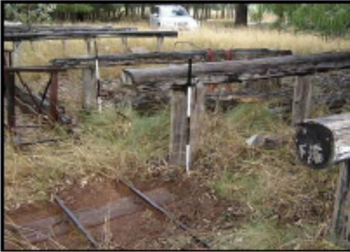
Plate 50 – View showing the differences in height between the first two rails and the third rail in the log rack (scales 1m).
